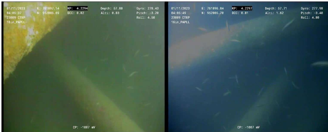
Figure 5 – 16" PAPLS pipeline Crossing Over 16" PAPLL at KP 4.233 (View from South)
