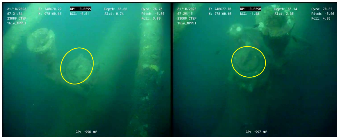
Figure 10 – NPPLI-Y1-16" Future (Blind) branch: Ball Valve . VB4 Indicator Open
