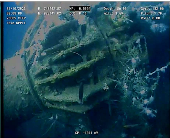
Figure 4 – (NPWI) NPPLI Riser Tie-in Flange KP 0.000 – Side view
