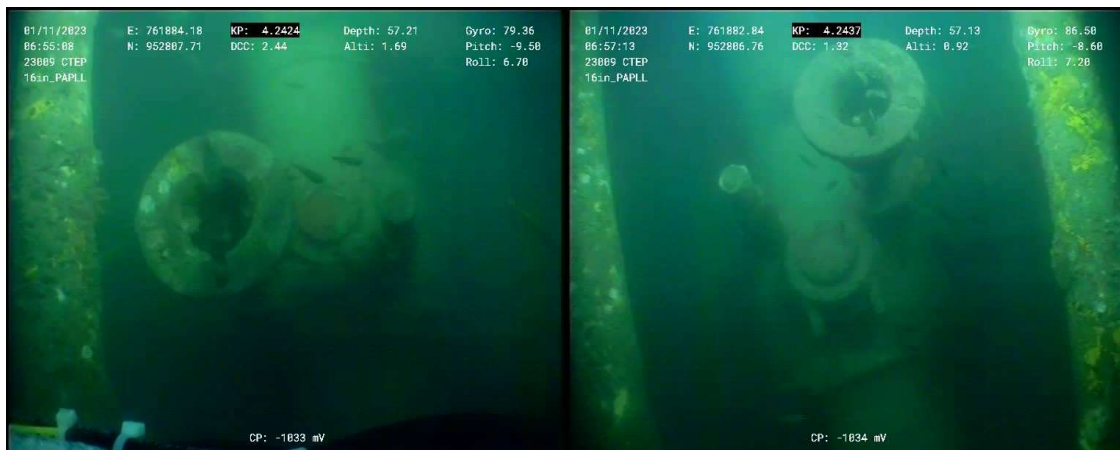
Figure 10 – PAPLL-Y1-16" PAPLL branch: Ball Valve - VB1 Indicator obscured
