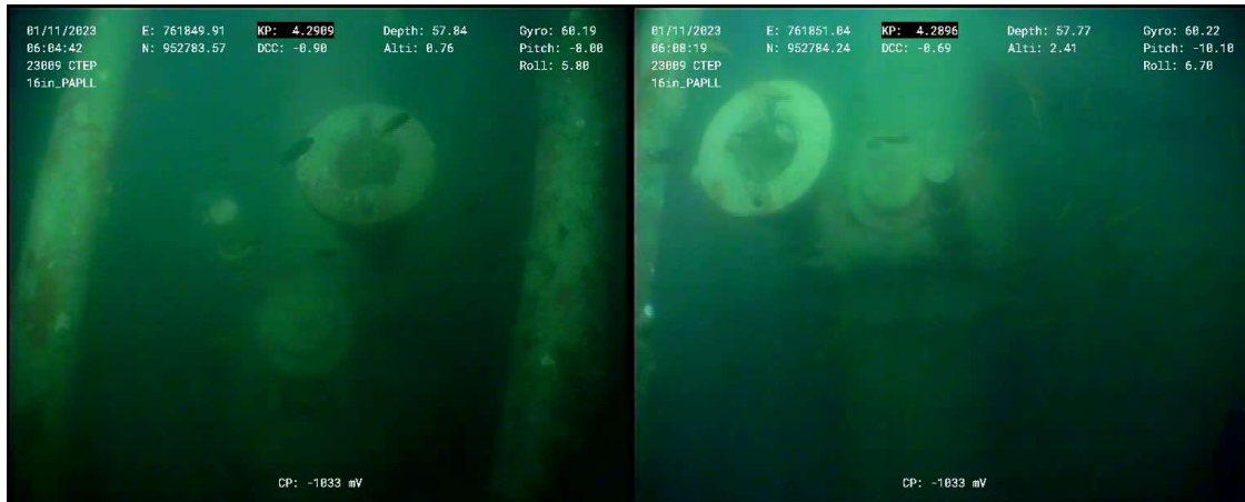
Figure 13 – PAPLJ-Y2-16" PAPLL branch: Ball Valve - VB3 Indicator obscured
