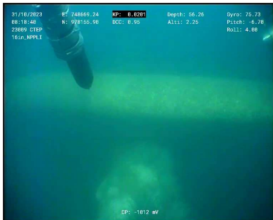
Figure 5 – Unknown pipeline Crossing Over 16" NPPLI at KP 0.021
