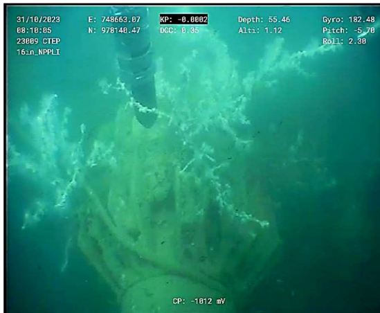
Figure 3 – (NPWI) 16in NPPLI Riser Tie-in Flange KP 0.000
