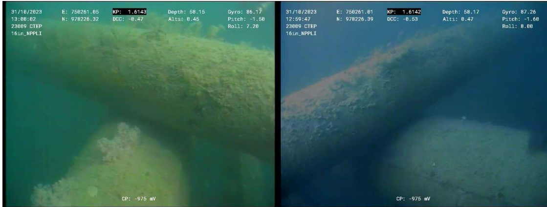
Figure 7 – Steel Sleeper supporting 16" NPPLI at KP 16.143 (view from North)
