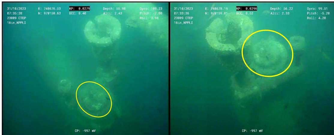
Figure 12 – NPPLI-Y1-16" NPPLI branch: Ball Valve . VB1 Indicator Open
