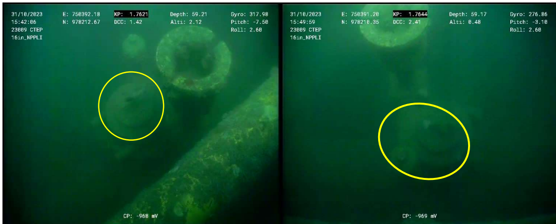
Figure 17 – NPPLI-Y2-16" NPPLI branch: Ball Valve . VB6 Indicator Open
