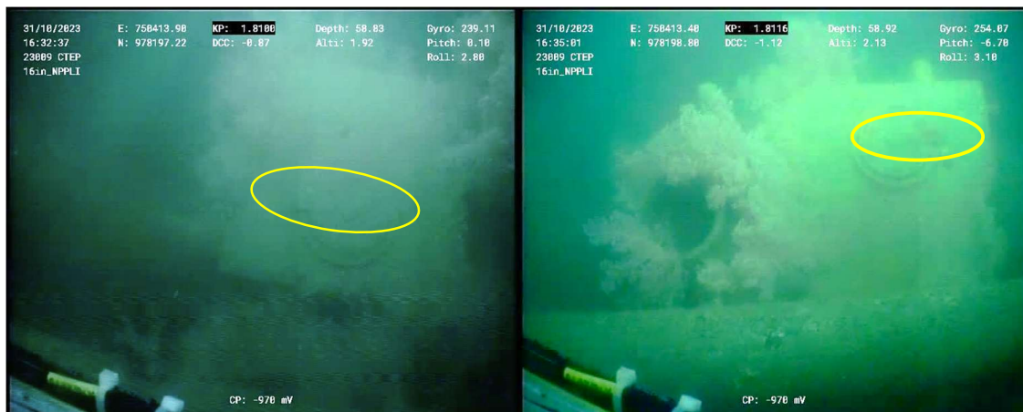
Figure 20 – NPPLC-Y1-16"NPPLC branch: Ball Valve . VB3 Indicator Open
