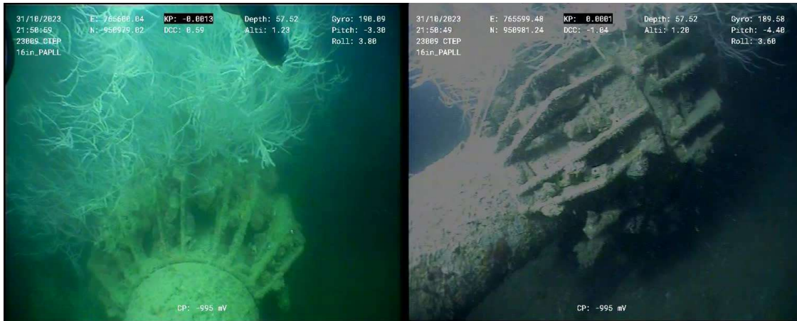
Figure 3 – (PAWL) 16in PAPLL Riser Tie-in Flange KP 0.000
