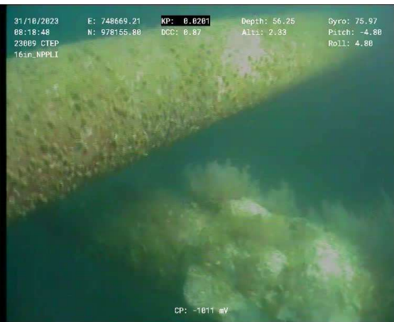
Figure 6 – Unknown pipeline Crossing Over 16" NPPLI at KP 0.021 (view from North)
